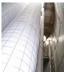
High Efficiency fibre Bed Mist Eliminator
